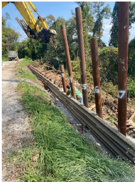
County Forces installing Pipe Piling Walls
