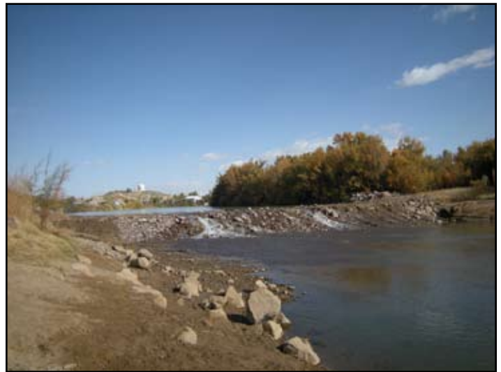
Figure 6.32. The Bureau of Reclamation seasonally constructs a temporary dam across the Rio Grande at the mouth of the wetlands at Rotary Park.
