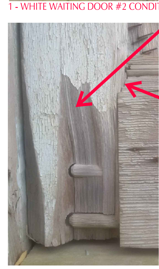
2 - WHITE WAITING DOOR #2 RAIL-STILE DETERIORATION 5 A-7 EXISTING DOOR CONDITIONS - FOR REFERENCE ONLY
