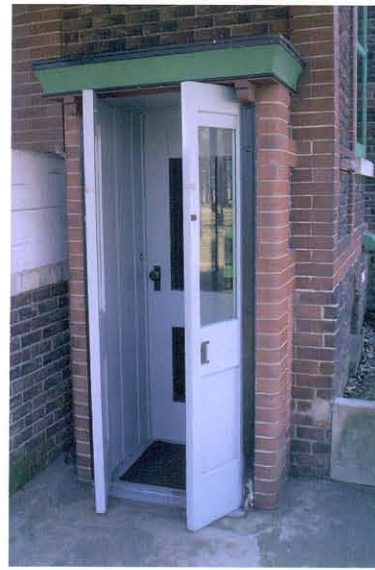
To keep out insects and other pests, Fred built automatically opening and closing entrance doors.
