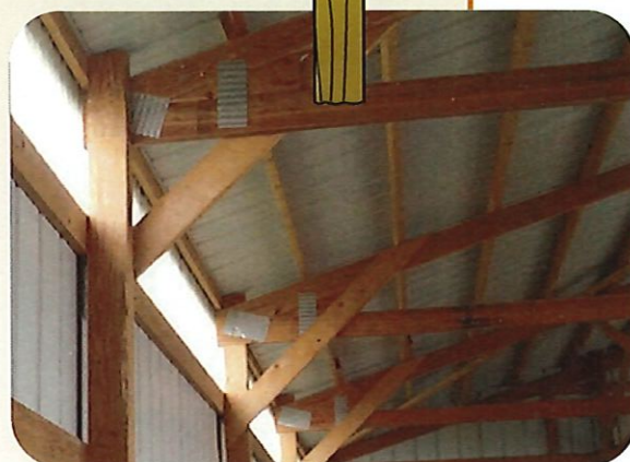
Weak Truss-to-Column Connection with 4 Foot on Center Trusses
