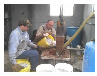
After determining our well depths we added rock and then placed 7 buckets of pelletized bentonite in the hole allowing it to settle to the bottom and set up for a couple of days before restarting the pump. The pump was re-started on Thursday at noon and ran continuous through Friday.
