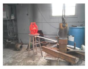
We lifted the test pump a few feet and moved it to one side of the casing allowing us to drop a marked mason line and plumb bob down the hole to determine what depth we were at without pulling the pump and bringing in a camera crew.
