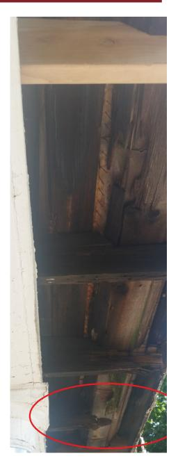
Picture of a recent project made possible by the Targeted Minor Home Repair Program. The project included replacement of rotted boards and repair of the front porch and will include painting the house, as well.
