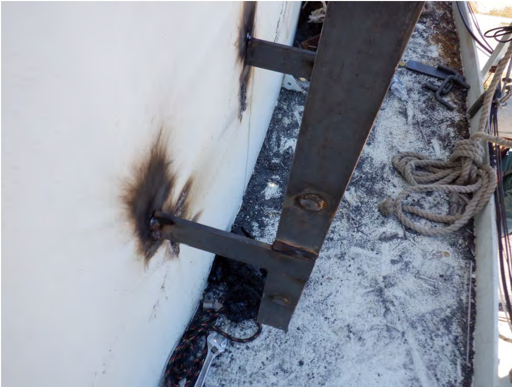
PHOTO #3: Bottom of the sidewall ladder with incomplete welds. All welds are to be fully seal welded and ground smooth.
