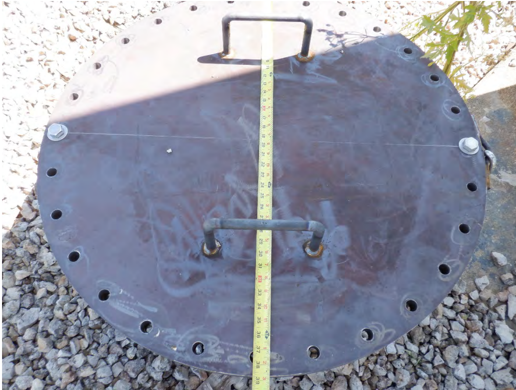
PHOTO #1: New 30" wet interior roof hatch does not have a hinge and does not match specifications of submittal drawings.
