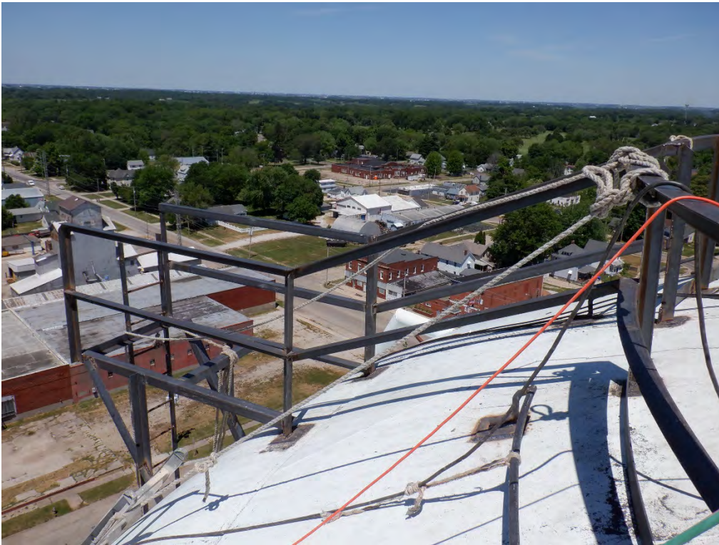
PHOTO #10: Sidewall ladder with step-off platform and safety rail.
