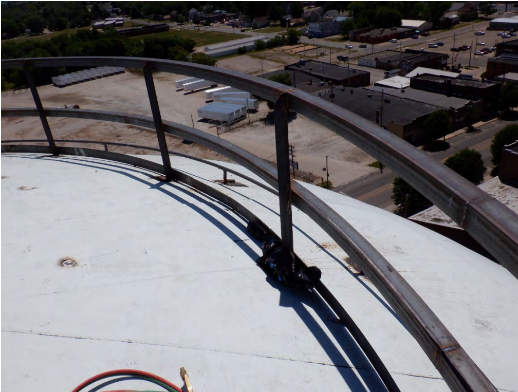
PHOTO #7: New roof safety handrail.
