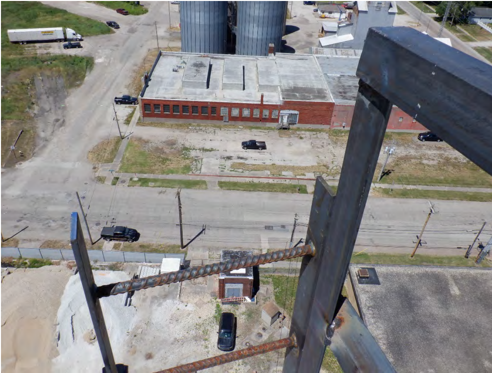
PHOTO #5: Sidewall ladder needs to be extended 12-inches to meet the top of the platform handrail.
