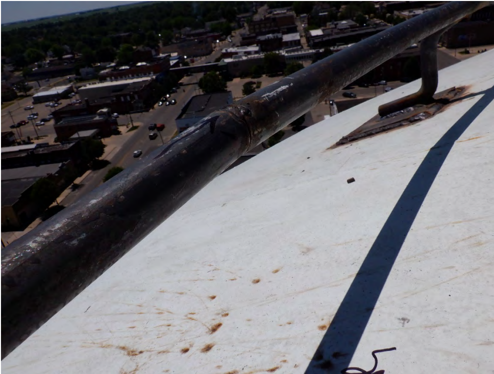
PHOTO #15: Painter's rail butt weld not located at a stand-off.
