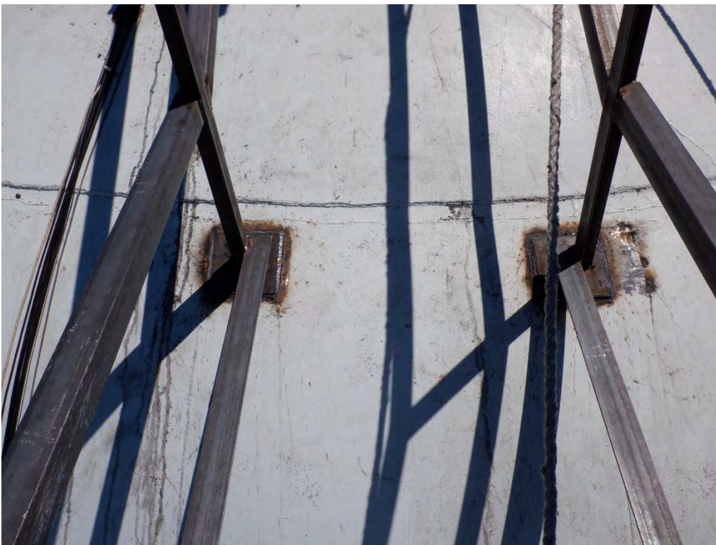
PHOTO #6: Step-off platform where platform and handrail meets the roof/knuckle. Stairs will be added to the roof to make the transition less steep.
