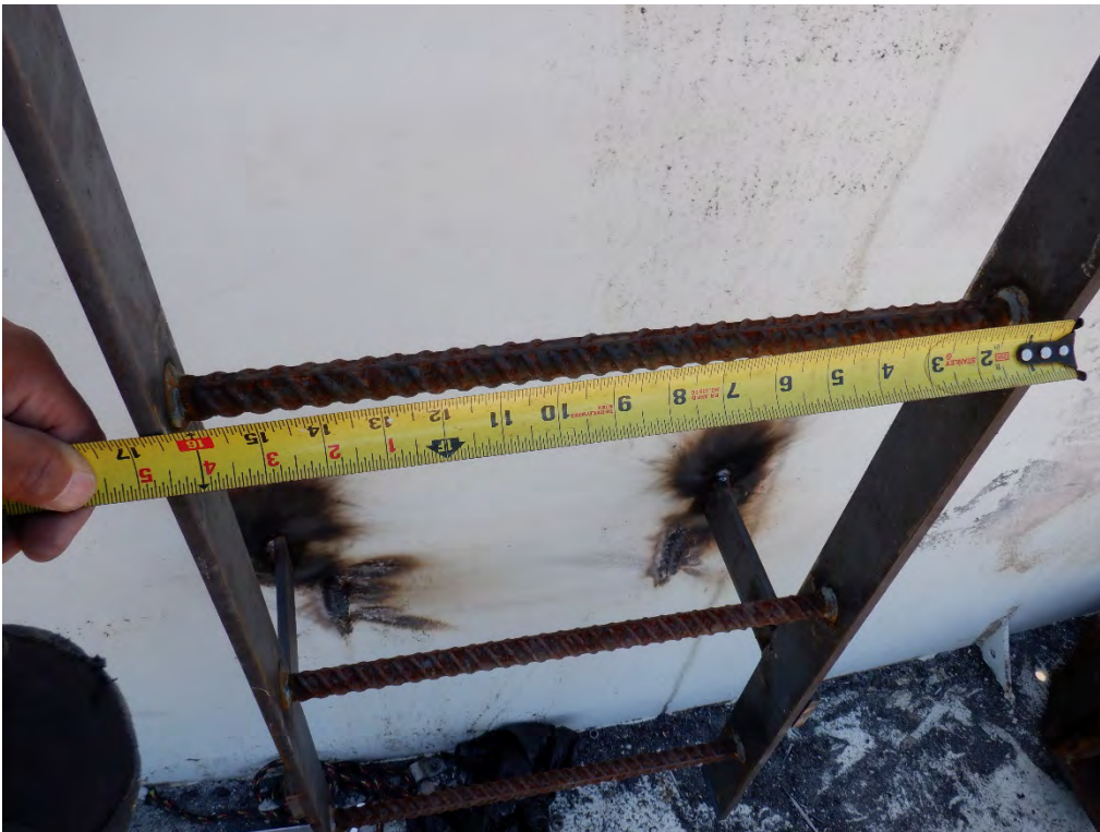
PHOTO #4: New sidewall ladder is 16" wide (inside ladder rails).
