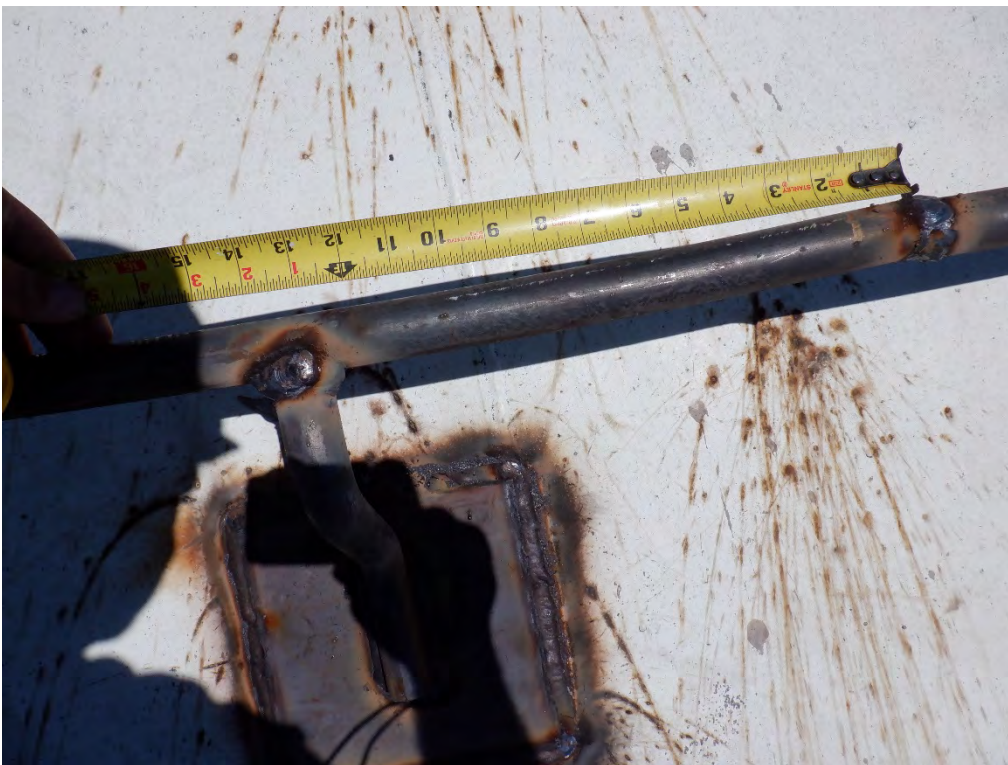
PHOTO #16: Painter's rail butt weld not located at a stand-off.
