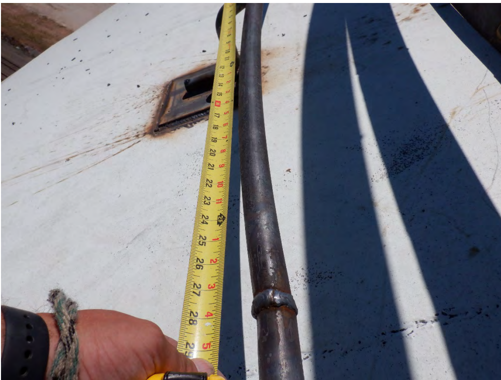
PHOTO #14: Painter's rail butt weld not located at a stand-off.
