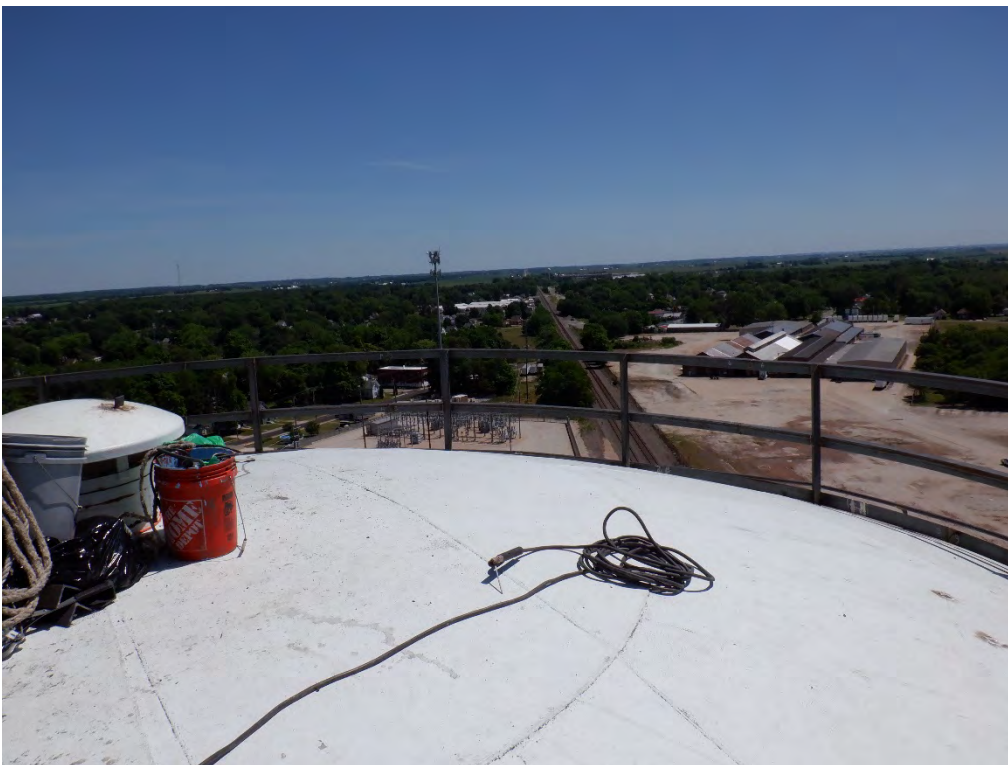
PHOTO #8: New roof safety handrail.
