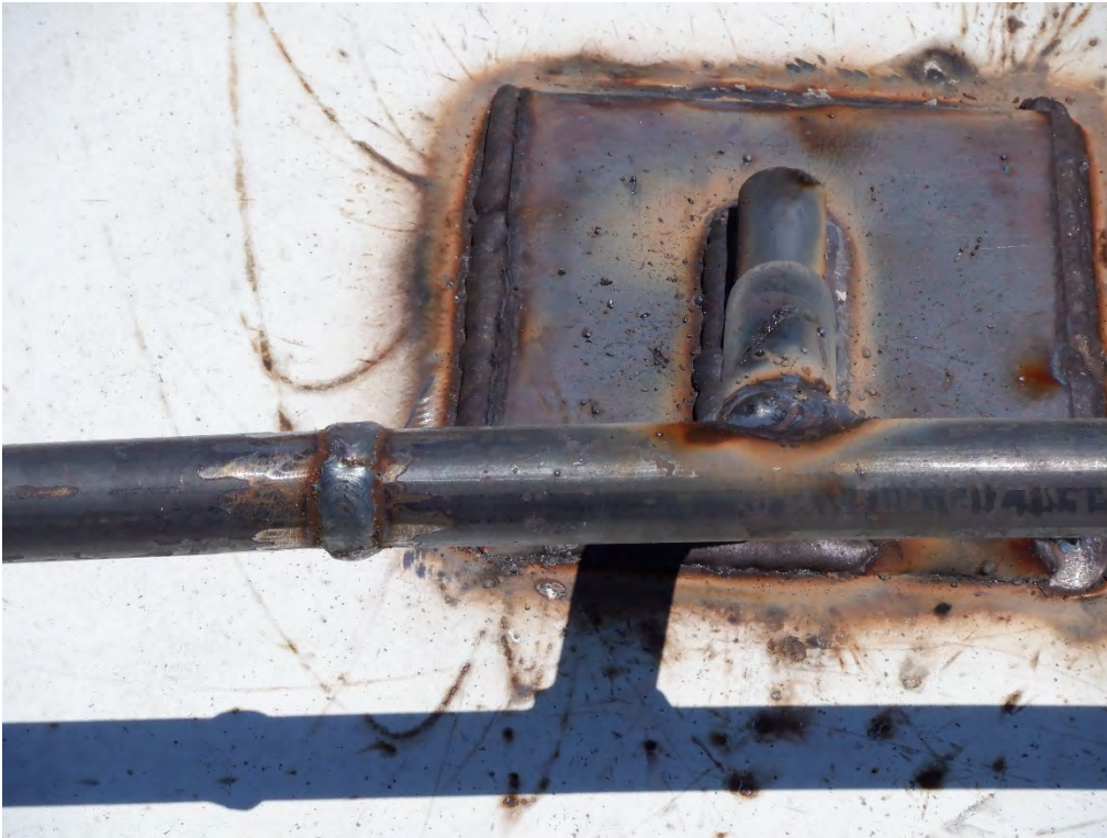
PHOTO #13: Painter's rail butt weld not located at a stand-off.
