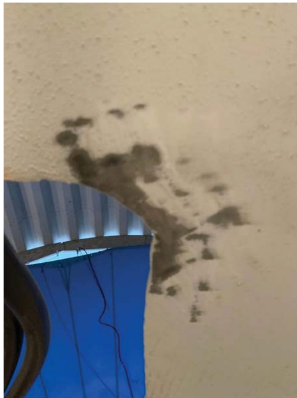
Spot power tool cleaning to the dry interior access tube.
