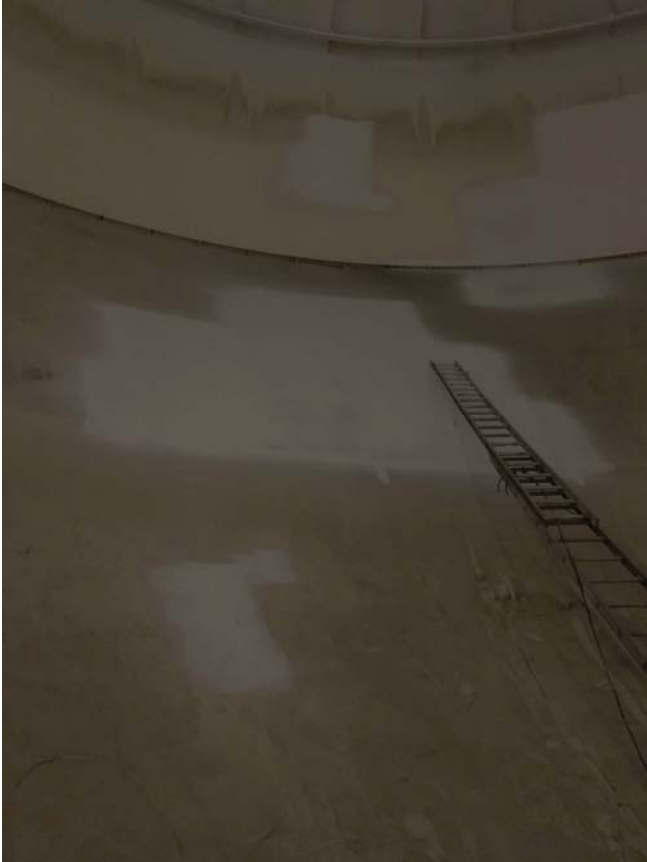
Topcoat applied to the wet interior bowl.
