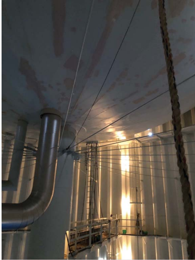
Prime coat applied to the dry interior bowl.
