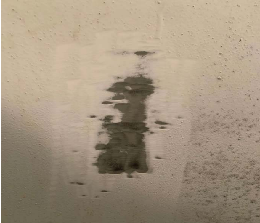
Spot power tool cleaning to the dry interior bowl.
