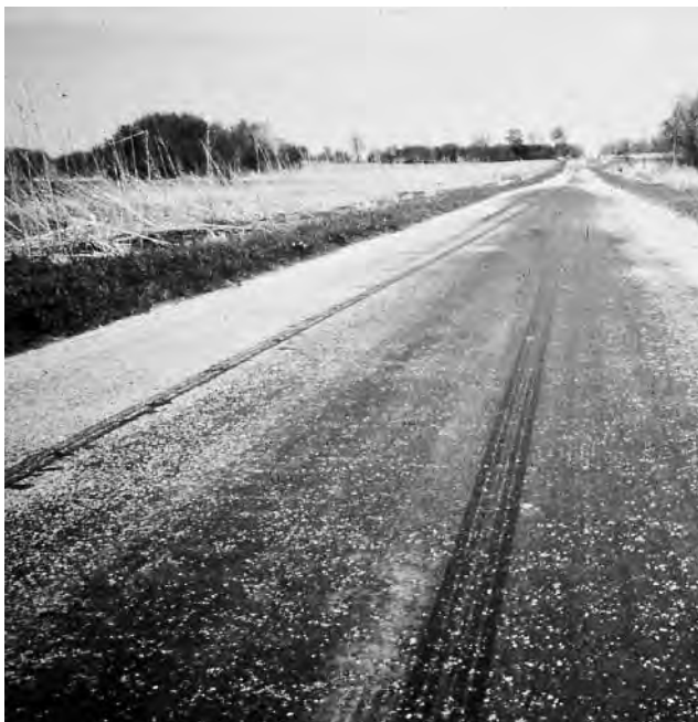
▼ Severe flushing.
