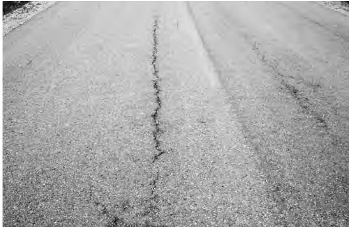
Multiple open, longitudinal cracks that are raveling. ▼
