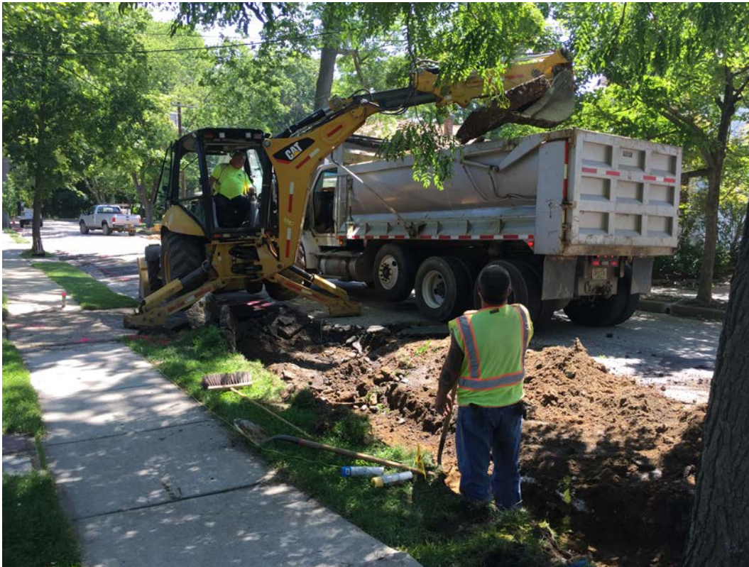
Removal of Concrete Curb on Springfield Terrace
