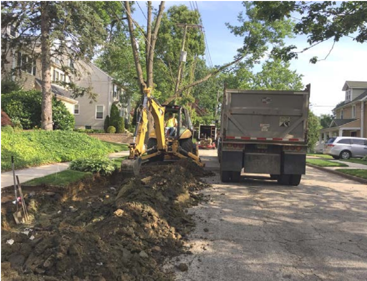
Removal of Concrete Curb on Walnut Street
