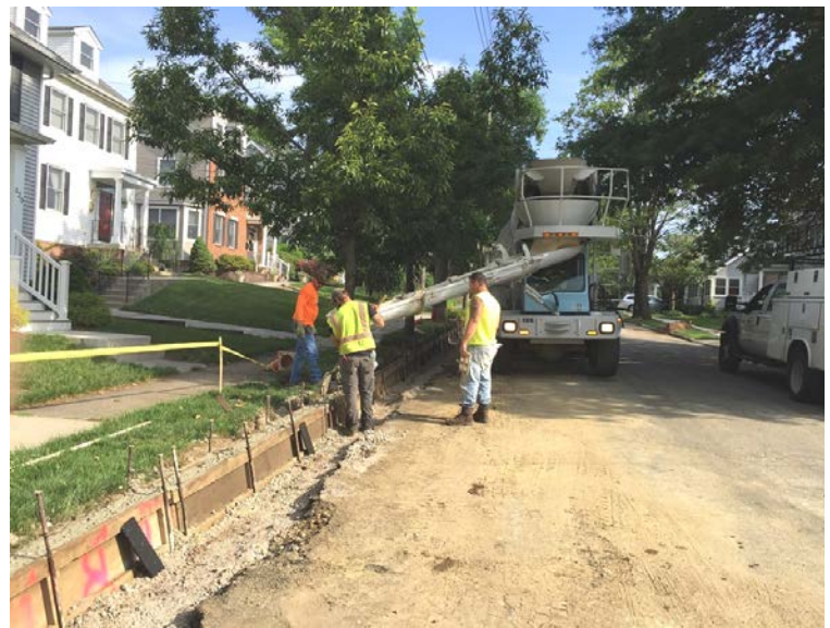
Pouring New Concrete Curb on Walnut Street
