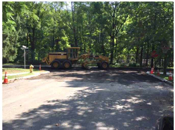
Grading Roadway Base on W. Atlantic Avenue at Mountwell
