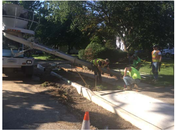
Pouring Concrete on W. Atlantic Avenue at Treaty Elm
