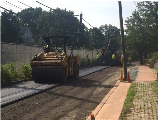
Final Paving on W. Atlantic Avenue Near Lincoln Avenue
