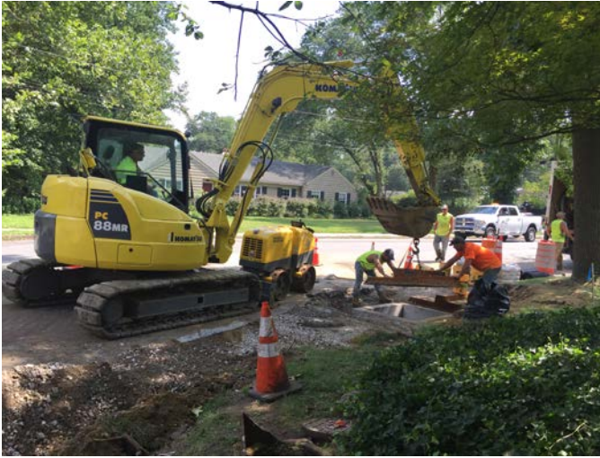
Installation of Drainage Inlet on Upland Way
