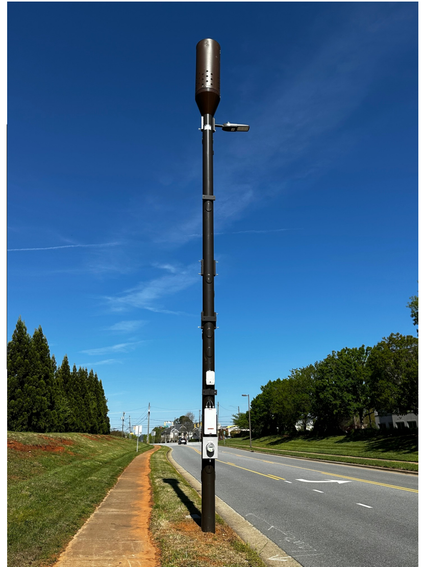
Concealed Small Cell Towers/Poles
