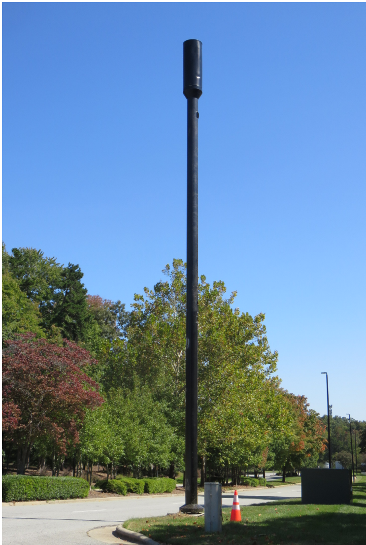
Concealed Small Cell Towers/Poles
