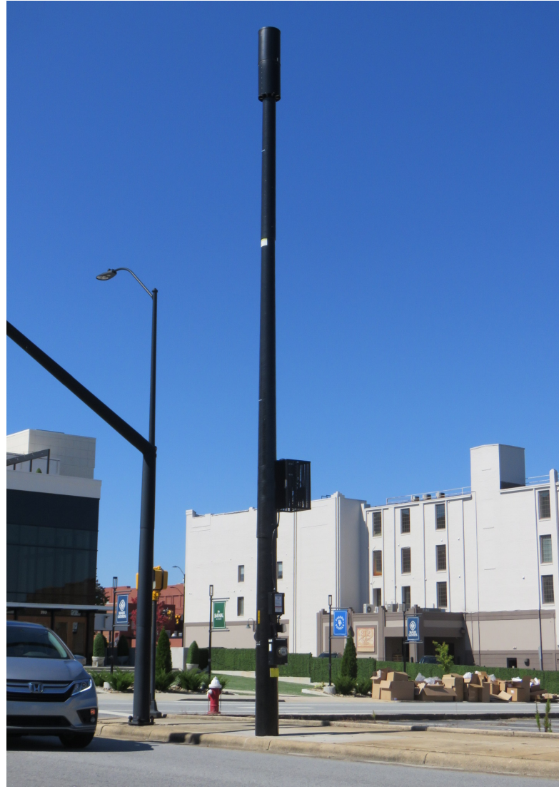
Concealed Small Cell Towers/Poles
