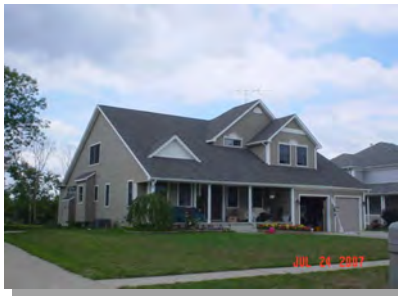
144600 24.14-2-21 162 Old Carriage House Rd
