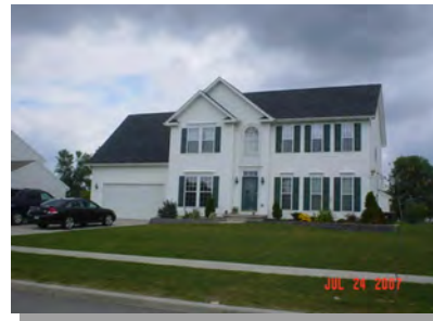
144600 24.14-1-47 79 Old Carriage House Rd
