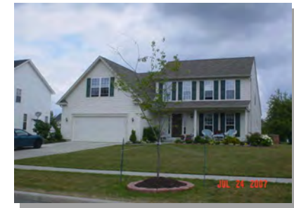
144600 24.14-1-48 71 Old Carriage House Rd
