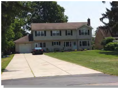
144600 23.06-1-12 4045 West River Pkwy
