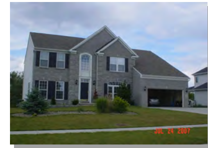
144600 24.14-1-38 98 Old Carriage House Rd
