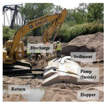
Figure 5. Installation of 30 ft long collector.
