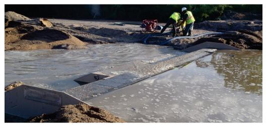
Figure 2. Sediment collector installed in Fountain Creek.
