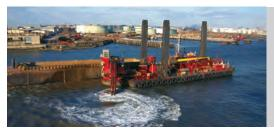
Maintenance dredging within the channels leading into the Port of New York/New Jersey was executed over eight contracts and multiple phases. Operations required deepening the channels from an original depth of 35 feet to 40 feet, then to 45 feet, and eventually to 50 feet.
