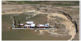
This project consisted of excavating material from a two-mile-long stretch of the Missouri River located along the Deer Island State Game Management Area in Iowa. The Rivers and Lakes team executed dredging efforts with the cutter suction dredge *Sandpiper* over a four-year, two-phase construction period. With a projected completion set for mid-summer 2014, this project focuses on creating shallow water habitats along the main channel border of the river. *Quantity*: 2.6 million cubic yards
