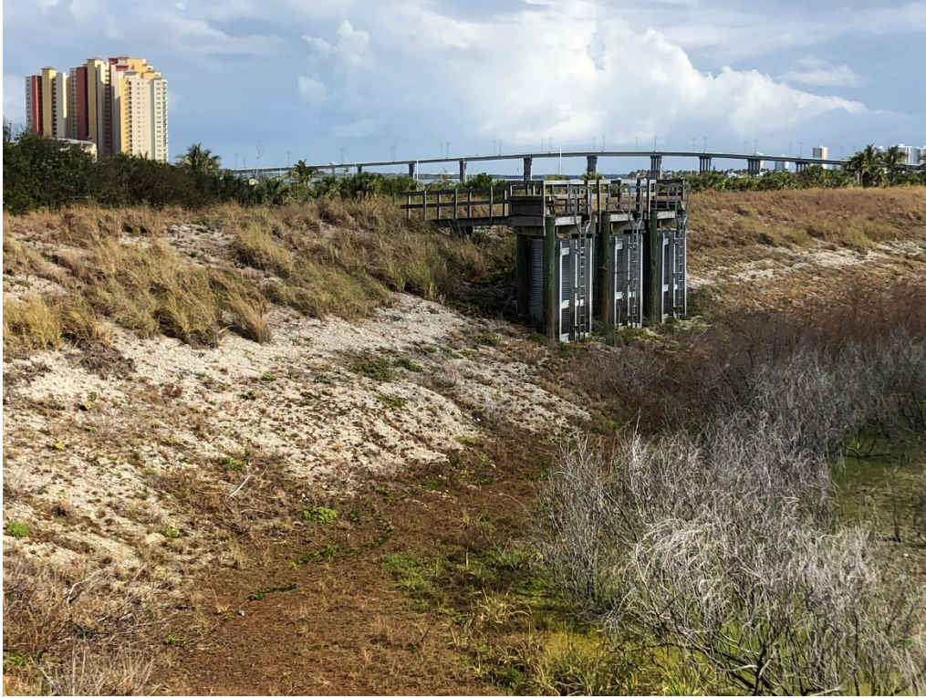
Photograph B5. Peanut Island DMMA half-pipe weir structure (looking northwest)
