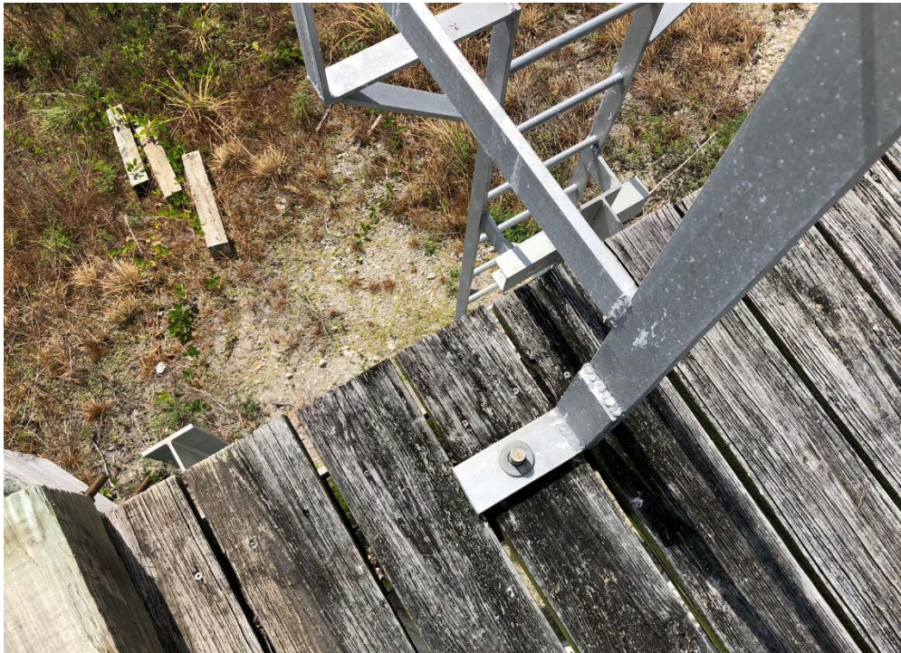
Photograph B6. Detail of weir ladder with missing nut
