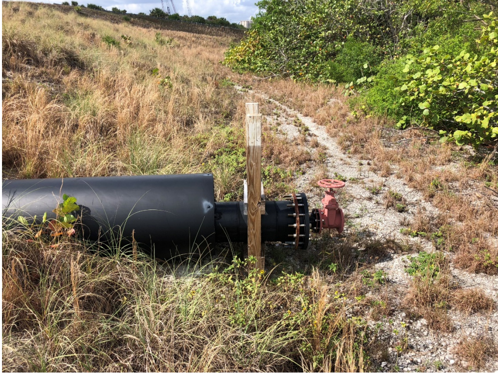
Photograph B11. Southernmost weir outflow pipe with gate valve (looking south)
