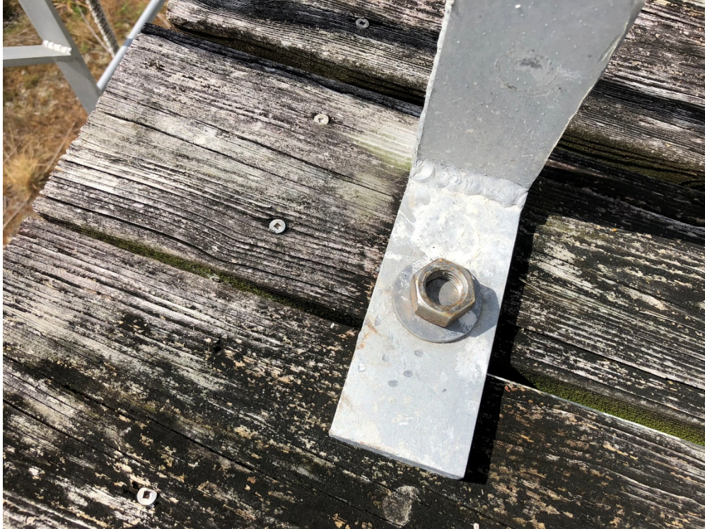
Photograph B7. Detail of weir ladder with loose nut
