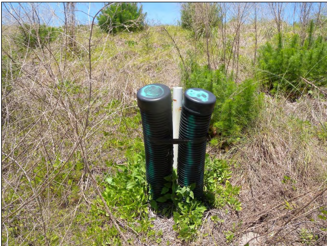
Image 4. View toward north of a wick drain outlet in southern stability berm
