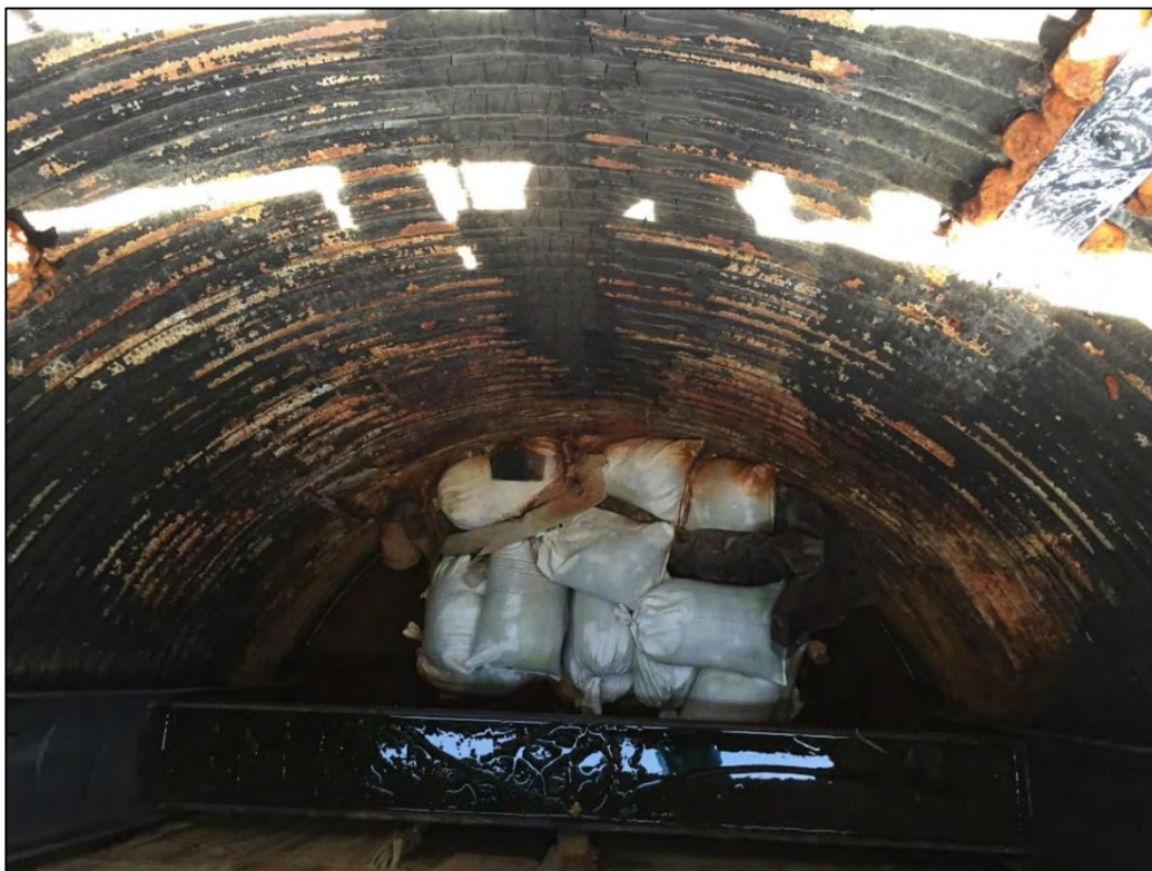
Image 18. Looking down into sandbag blocked weir #1 inlet. Weirs 2, and 4 are in the same condition
