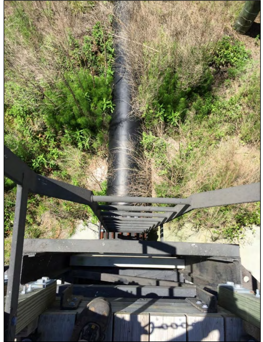
Image 12. Looking down at HDPE weir outlet pipe prior to its crossing through the western dike
