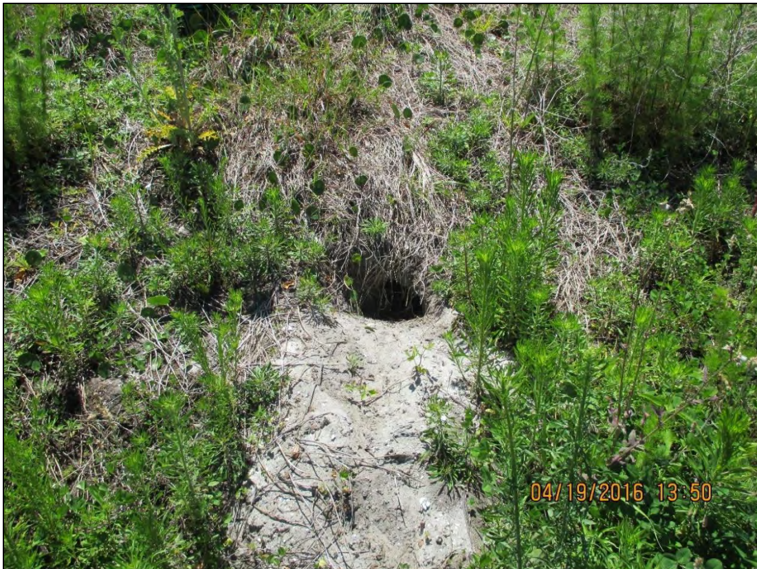
Image 20. Animal burrow into eastern stability berm
