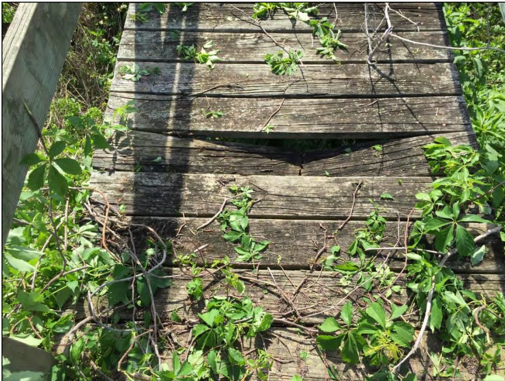
Image 15. Broken board on weir walkway timber deck
