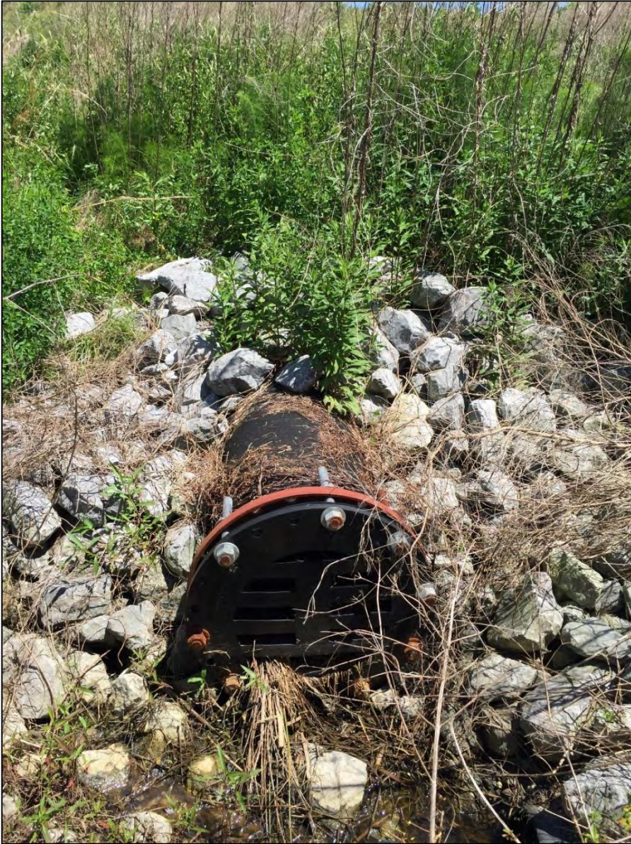
Image 15. Looking east at flanged end of weir outlet pipe
