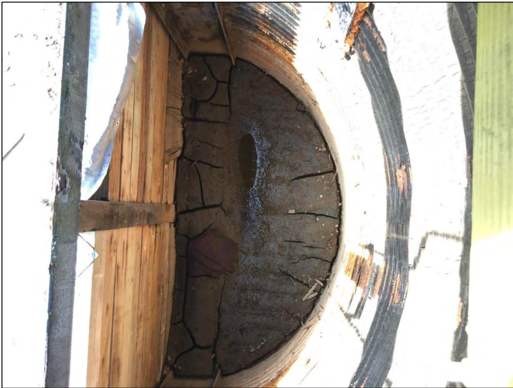
Image 17. Looking into weir #3 at sediment blocking inlet
