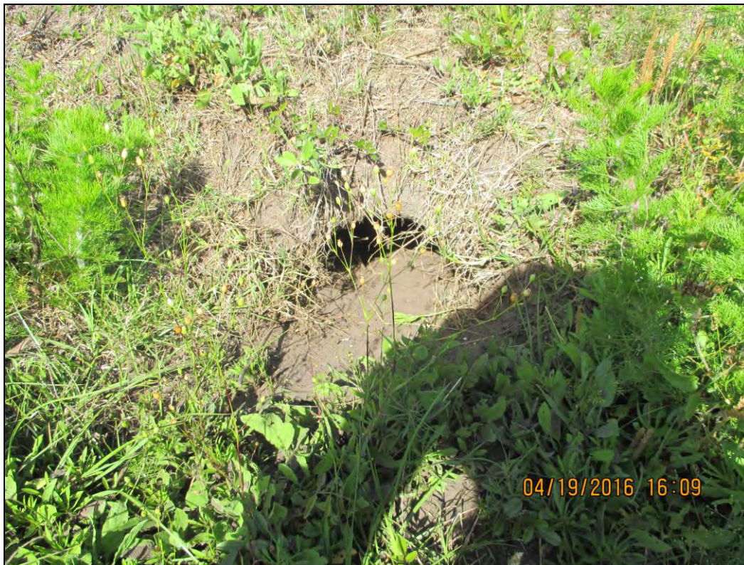
Image 31. Looking east at a gopher tortoise burrow into the exterior of the southwestern embankment
