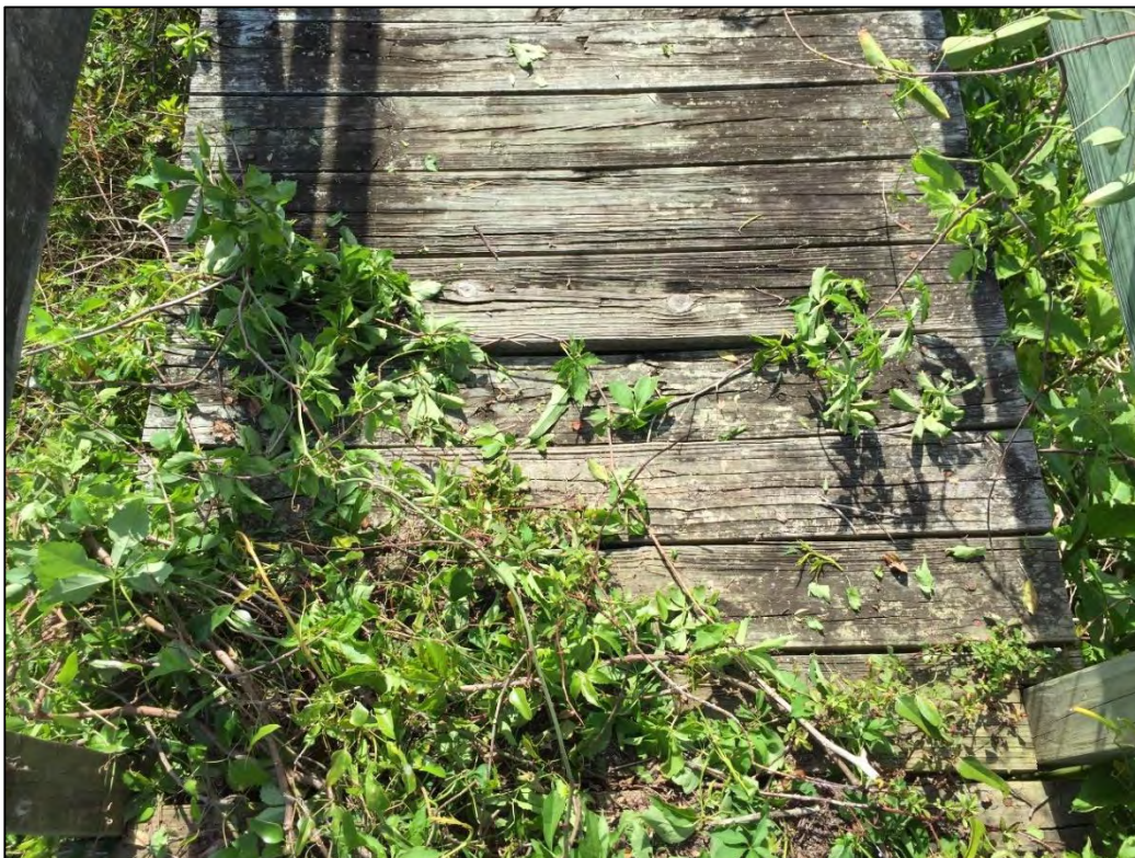
Image 16. Broken, decaying, board on weir walkway timber deck
