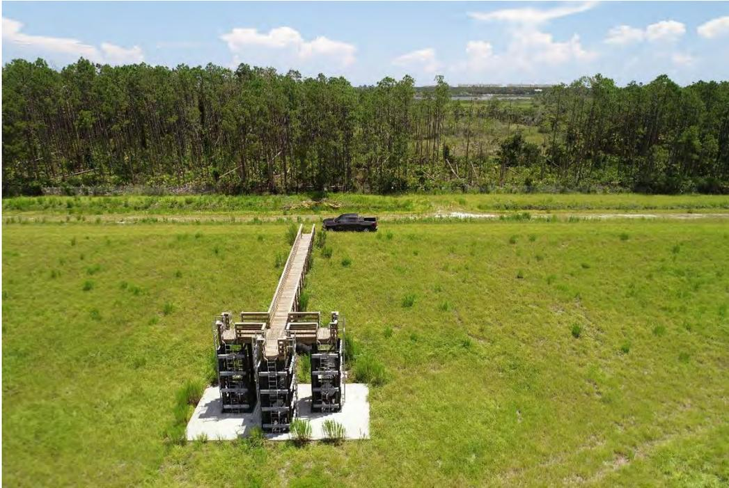
**Image 9.** View looking east, toward the waterway, of weirs and timber deck walkway.
