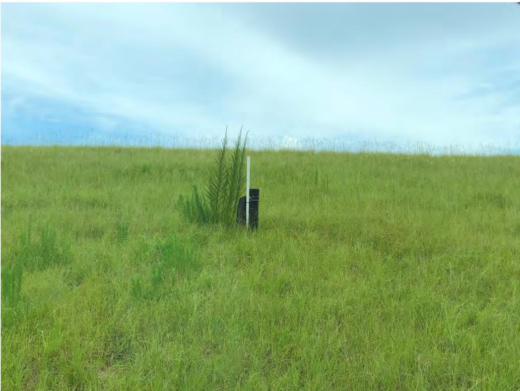
**Image 4.** View toward north of a toe drain outlet in southern stability berm.
