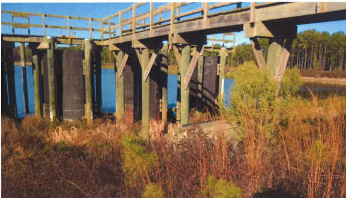
Photograph B11. DMMA DU-9 timber weir deck and weir structure (looking northwest)
