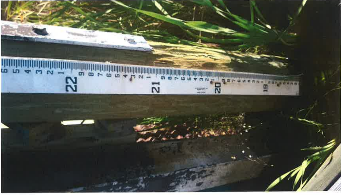
Photograph B14. Pile rot on exterior and gauge
