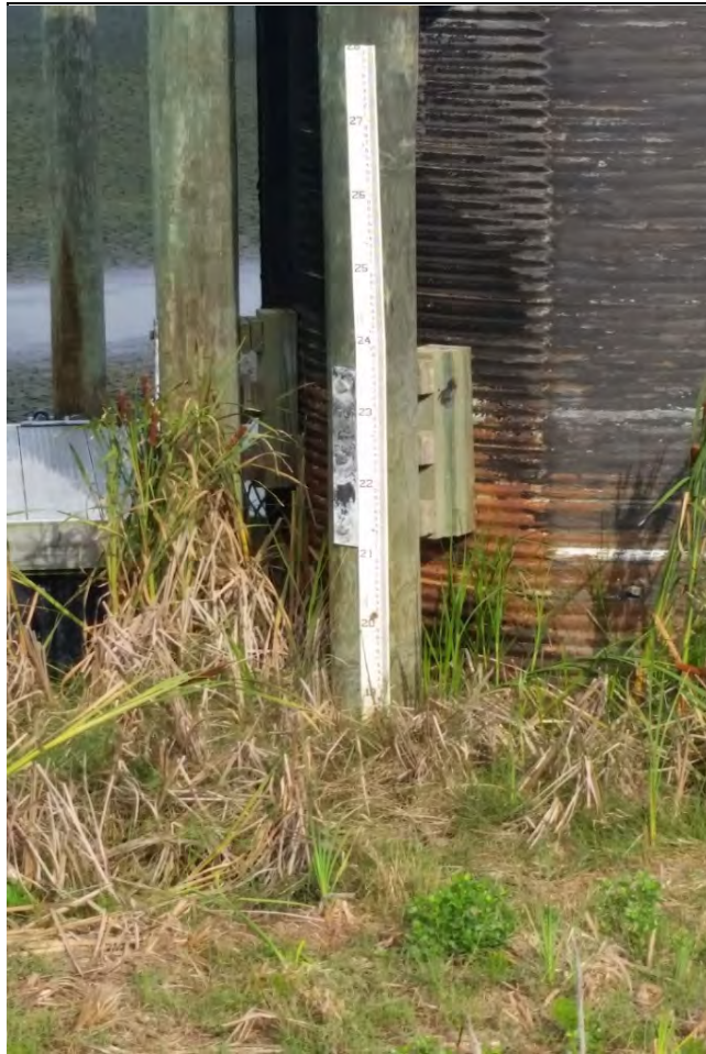
Photo 16: South side of weir structure, showing depth gauge.
