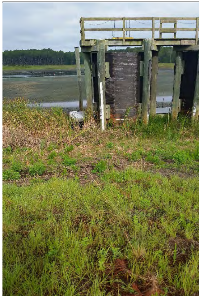
Photo 15: South side of weir structure, showing depth gauge.
